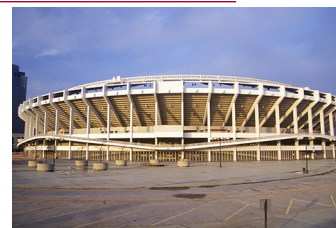
William Hughes '66 helped develop steel components for the construction of Three Rivers Stadium, Pittsburgh.
